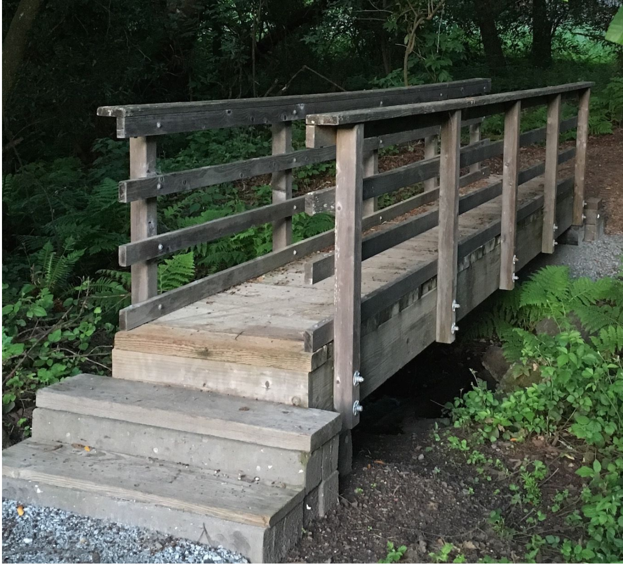
New Pedestrian Bridge Connecting Camp Area to Bathroom
